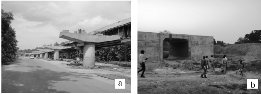
Fig. 5. (a) A over pass designed for wildlife crossing in the Pench-Kanha Corridor (b) A culvert designed for movement of smaller fauna
